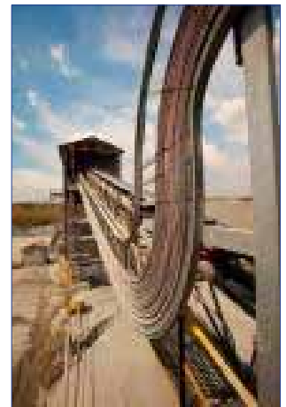
Right: New cable rack installed
